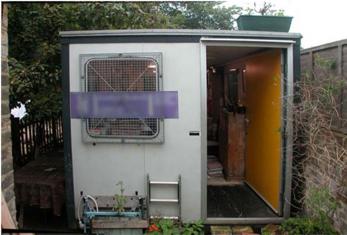
Figure 26. 'Live-nearby' (building surveyor), London borough, 2005
